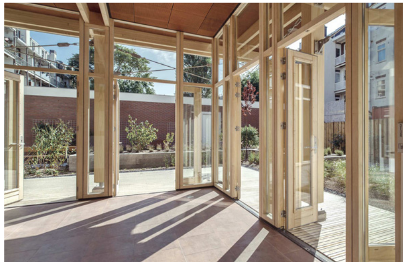
FagelCats - Accoya Structural used for apartments and care complex for elderly people in Amsterdam // www.accoya.com
